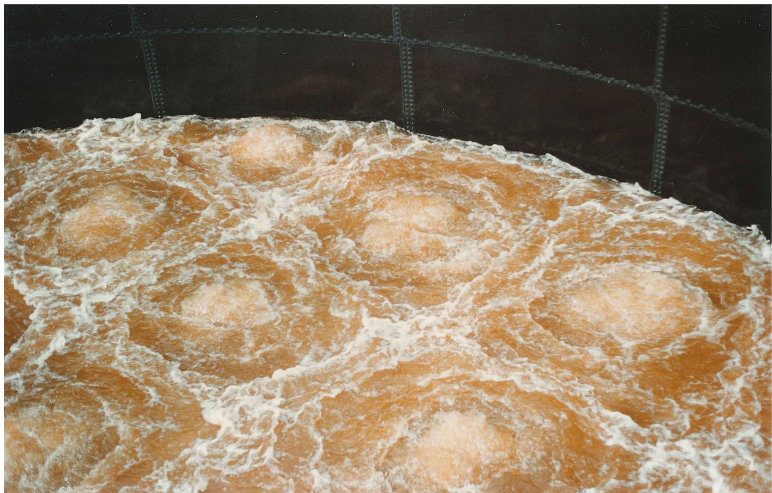
Picture 7: optimal aeration and mixing
