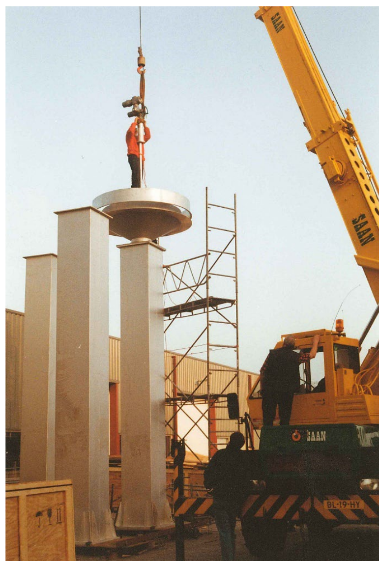
Picture 4: skimmer for a 625 m 3 /h plant
