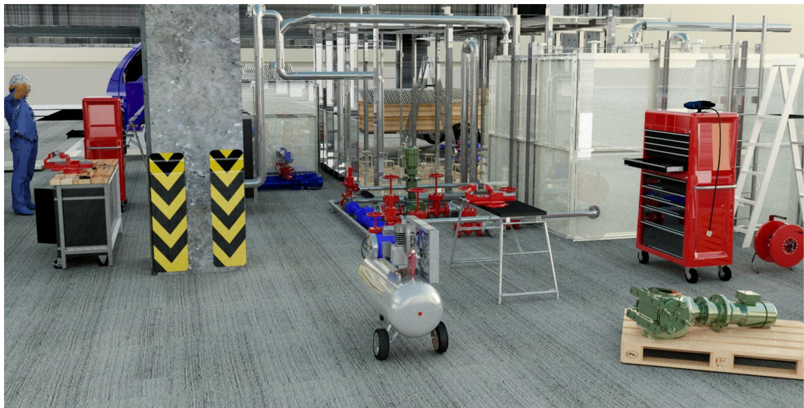
Picture 3: modular sewage treatment plant installed in the basement of a building
